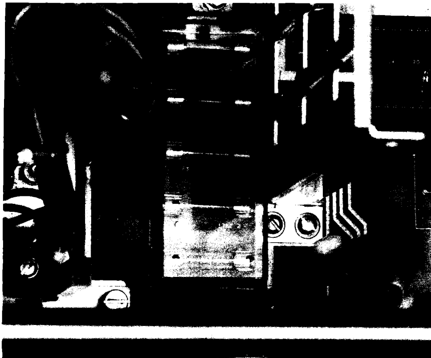
Figure 8-23. Secondary Fuse Area
